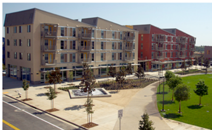
UC Davis West Village is a mixed use community that includes approximately 42,500 square feet of retail space on the perimeter of a Village Square that has been designed as a hub of neighborhood activity. (Karin Higgins/UC Davis photo)
